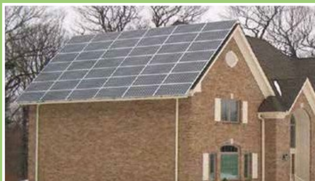
Typical retrofit. Note: No clearances along edges
